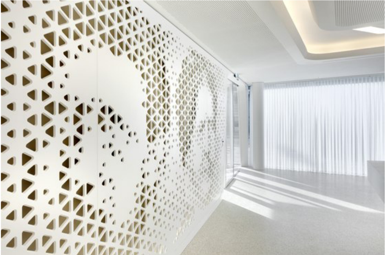
The detailed pattern was created using digital processes and then cut by a CNC milling machine; photo: Jan Bitter
