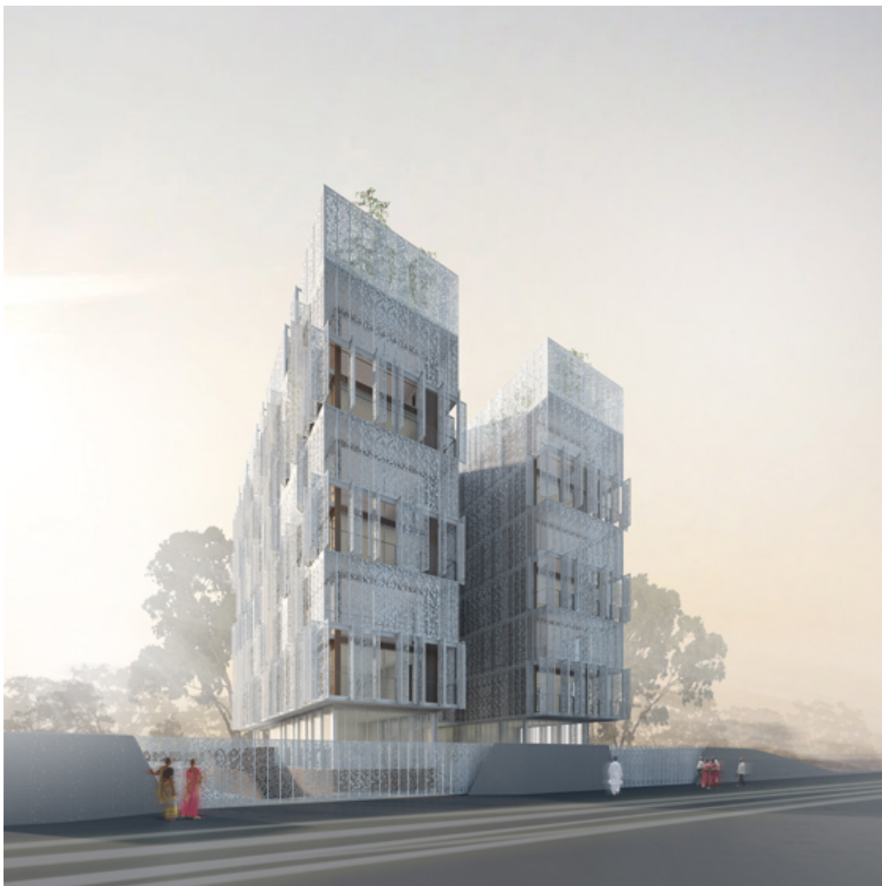
The perforated steel façade of Piercy Conner Architects' Restello apartment building provides natural ventilation and shade; image © Piercy Conner Architects
